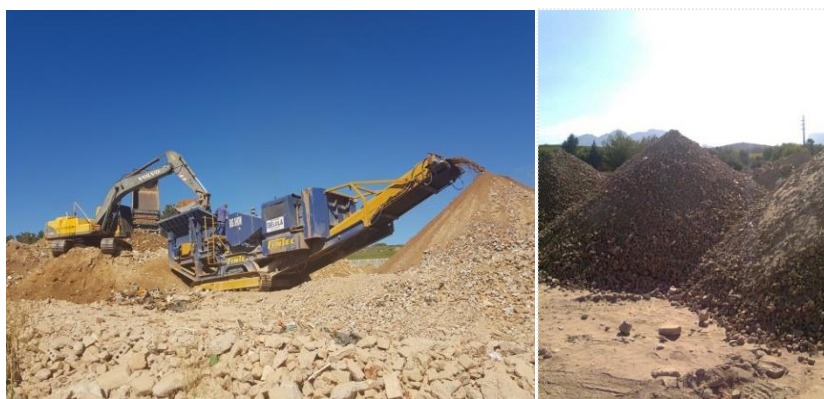
Rubble crushed and screened on site Crushed stone stockpile
